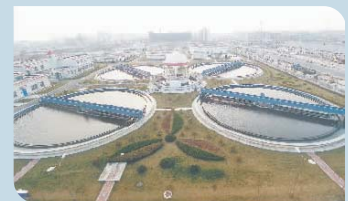
Huai-an Sewage Disposal Plant in Jiangsu Province
