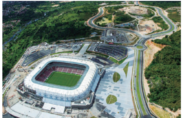
Itaipava Arena Pernambuco under construction
