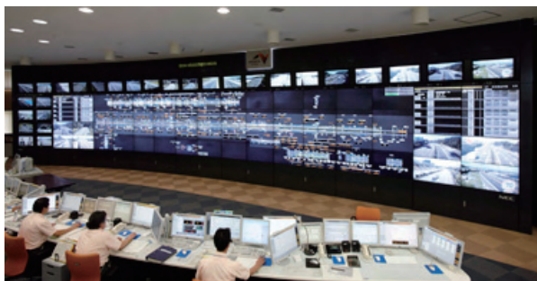
The giant screen at the control center
