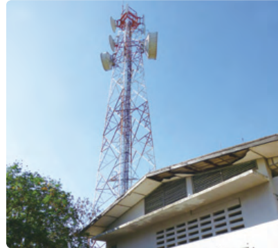
NEC has received an order for a core optical transmission network in Myanmar
