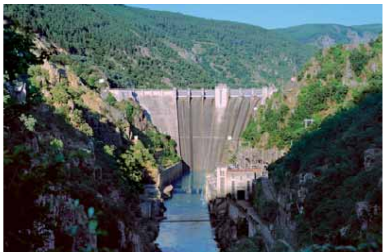
Hydroelectric plant at San Esteban (Ourense).
