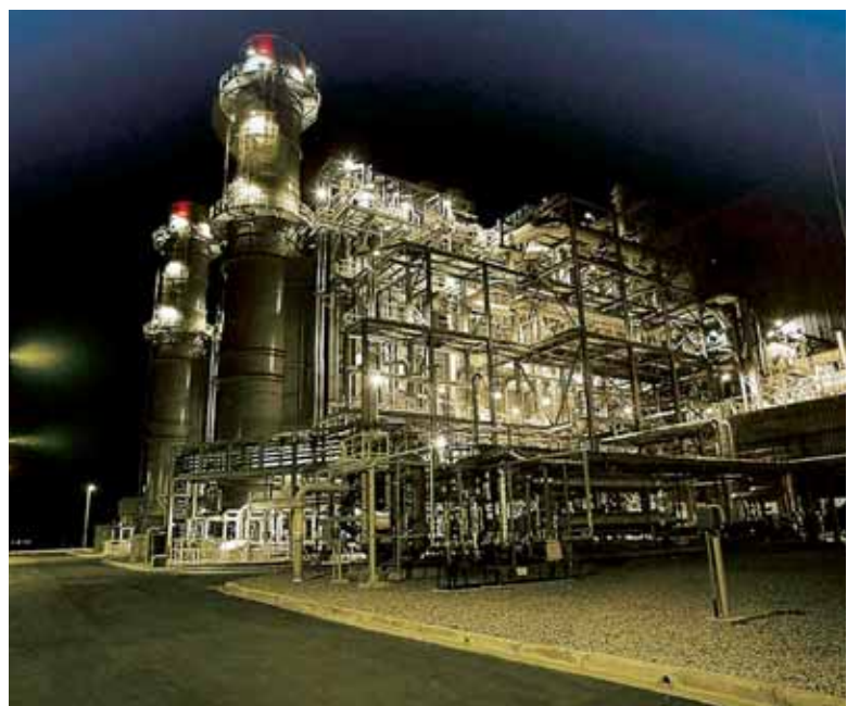
Combined cycle plant at Termopernambuco, Brazil.
