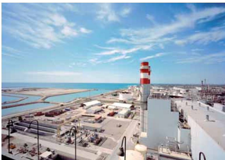
The Castellón combined cycle power plant.
