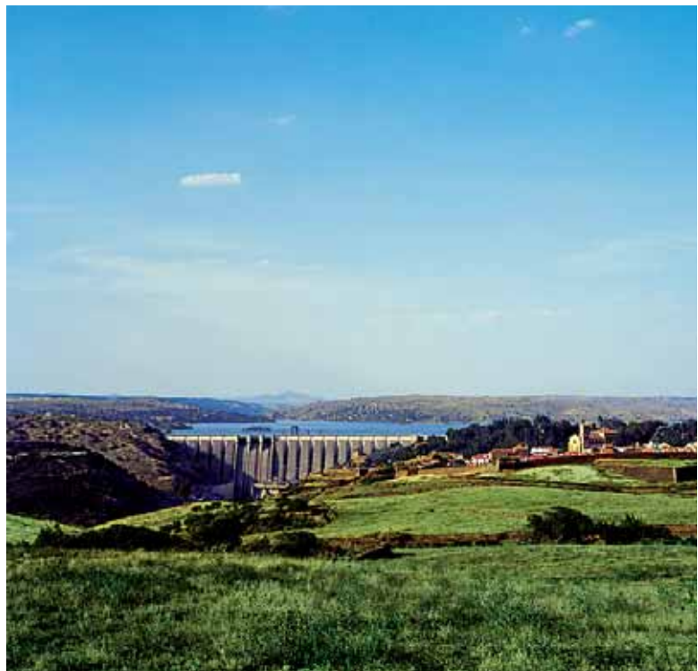
José María Oriol hydroelectric plant in Alcántara (Cáceres).
