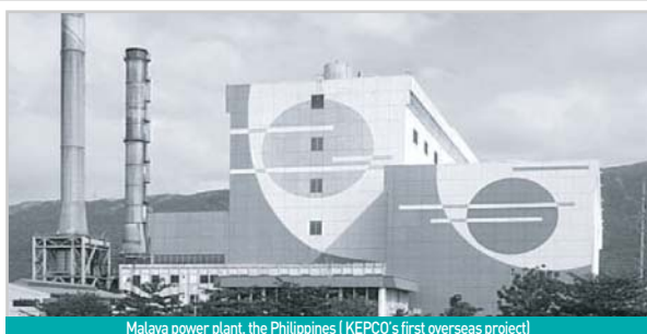
Malaya power plant, the Philippines | KEPCO's first overseas project
