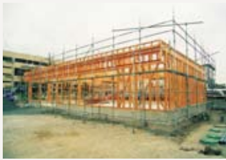
Store under construction
