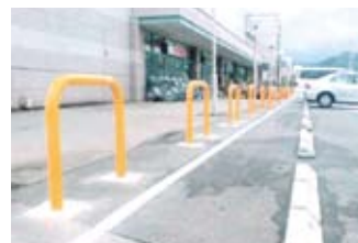
Parking Lot Guardrails
