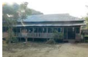
Old school building in Myanmar with no walls
