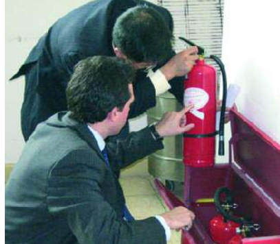
2 Inspection of safety equipment
