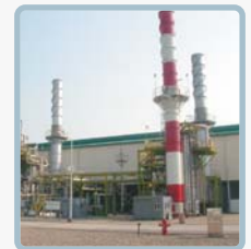
Cogeneration power plant
