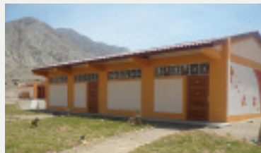
Restored school in Peru
