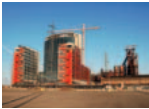
The building of Dexia Bank in Belval, Luxembourg
