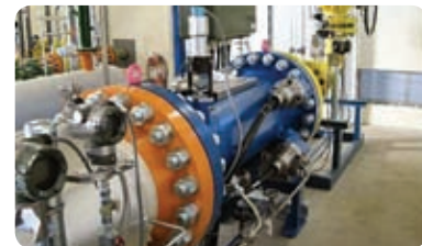
▲ Generating Equipment Using Gas Pressure
