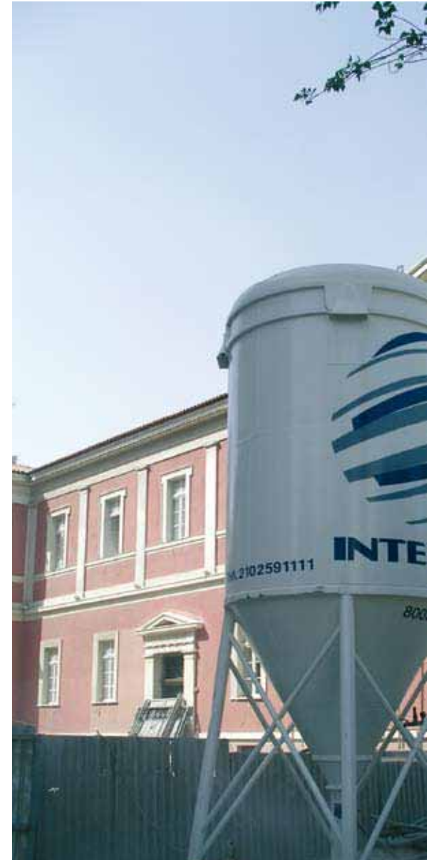
Construction and renovation of Law School, Athens, Greece, 2006
