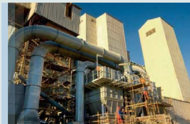
New dust extractor at the Sasol Nitro fertiliser granulation plant.
