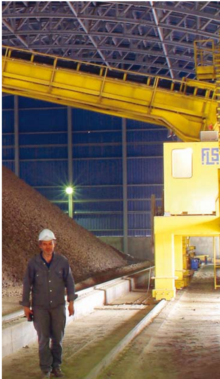
Prehomogenization of raw materials area, Thessaloniki - Greece, 2005
