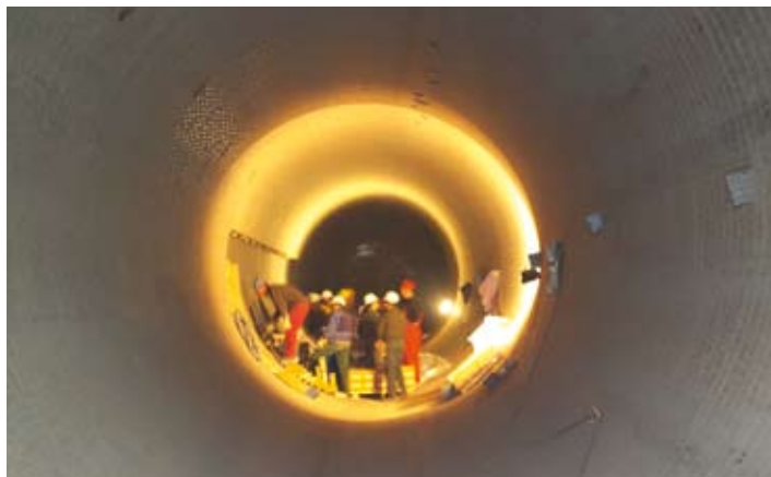
Kiln lining repair, Kamari plant - Greece, 2005
