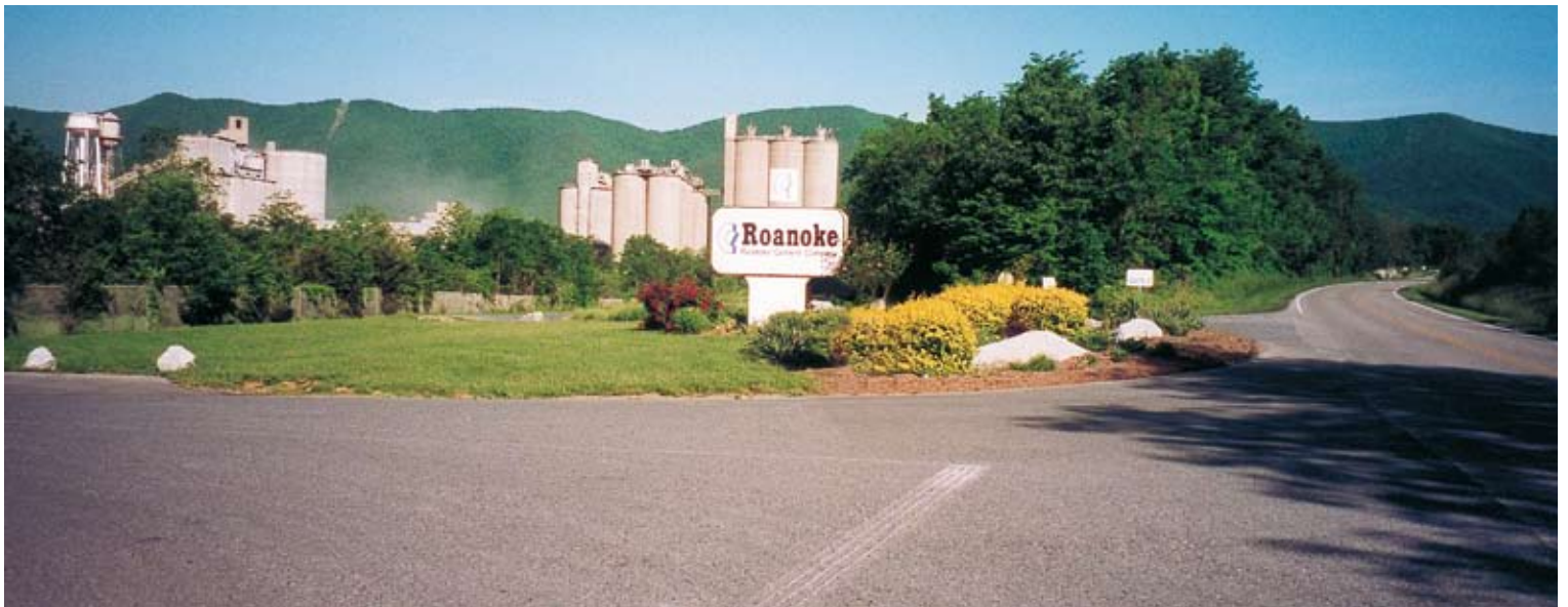
The Roanoke plant – USA, 2005
