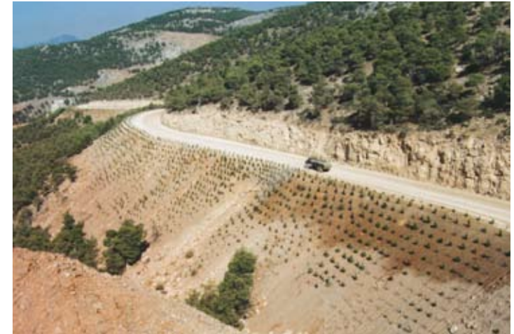
Rehabilitation of Xirorema quarry – first stage
