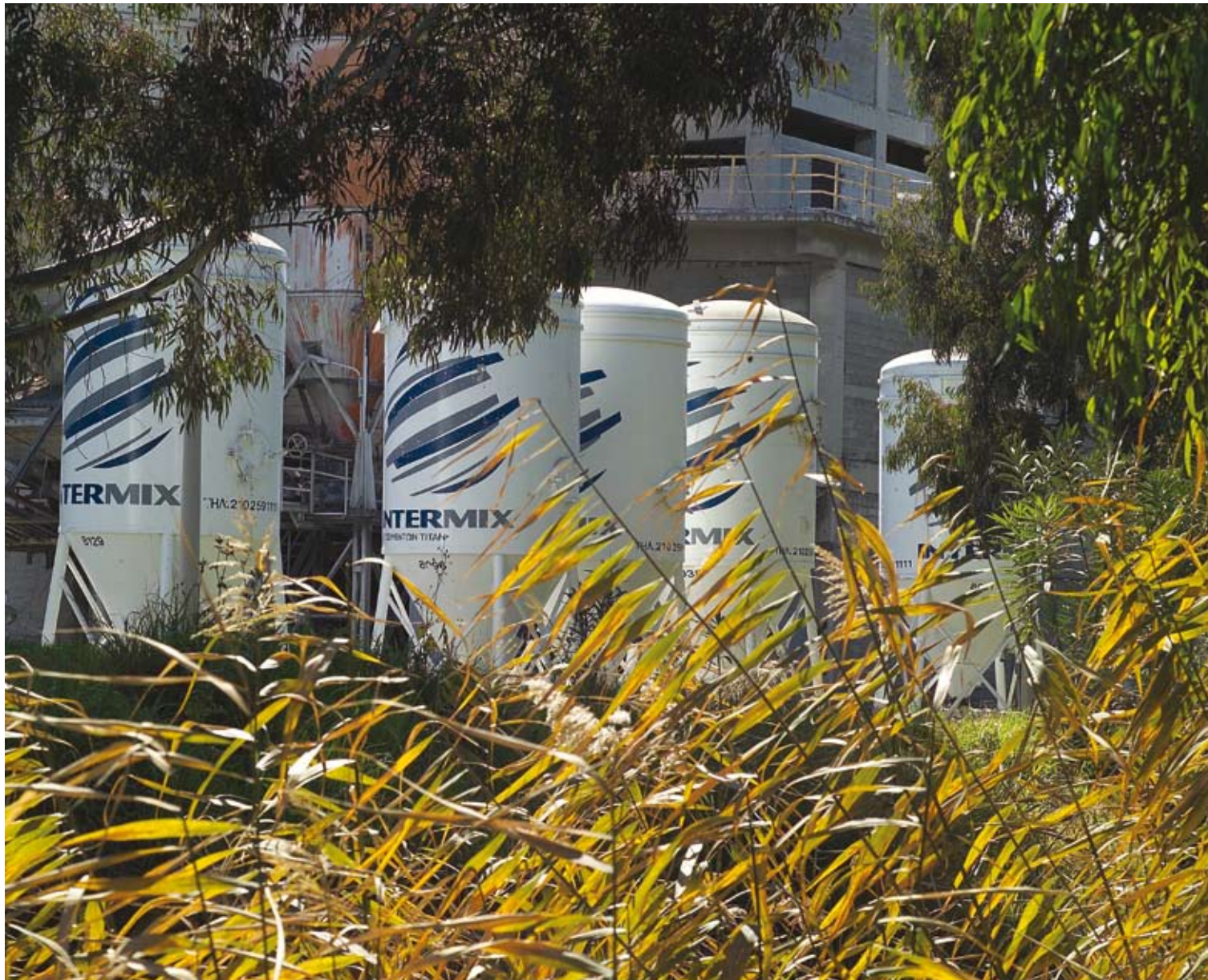
Dry mortars facility, Eleusis - Greece, 2005
