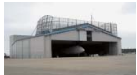
Noise reduction hangar at Narita Airport
