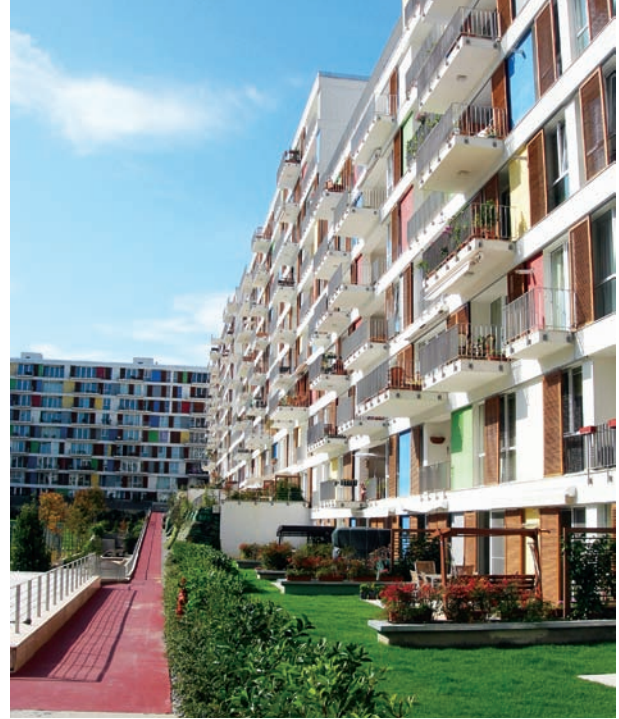
Evidea Residential Project in Çekmeköy
