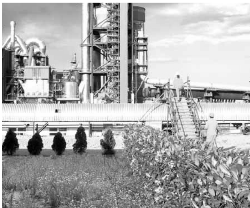
Antea cement plant, Albania
