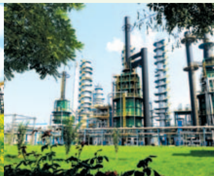
The refinery of Sinopec Cangzhou Company, located on a once-to-be alkali flat
