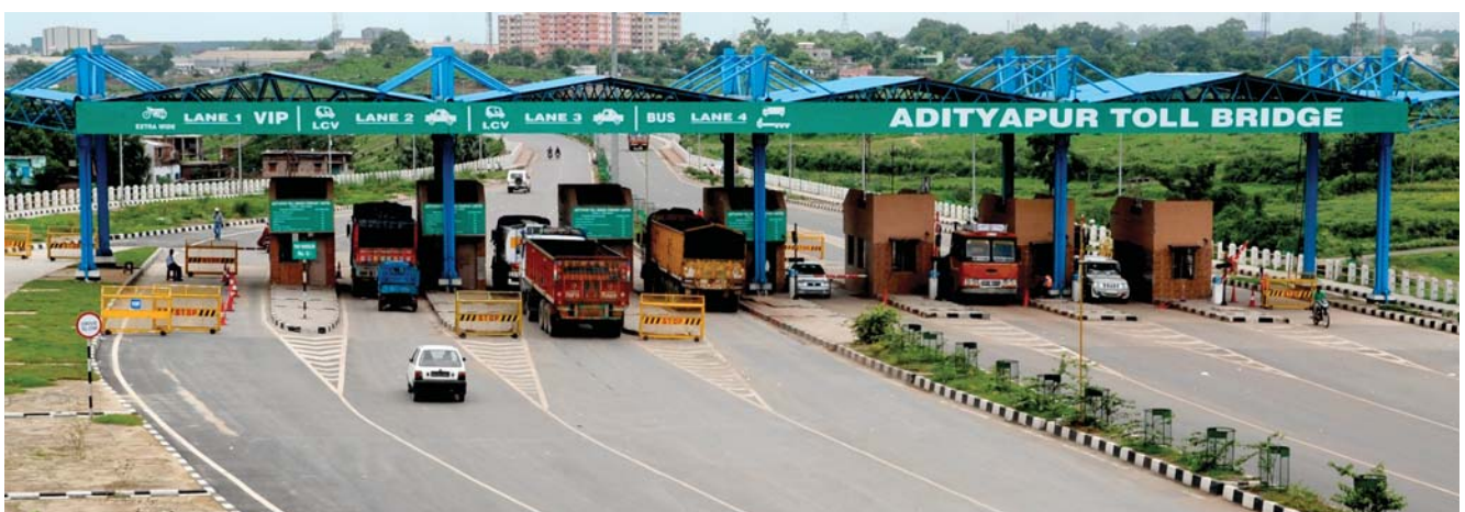
Adityapur Toll Bridge was built and is now managed by subsidiaries of Tata Steel
