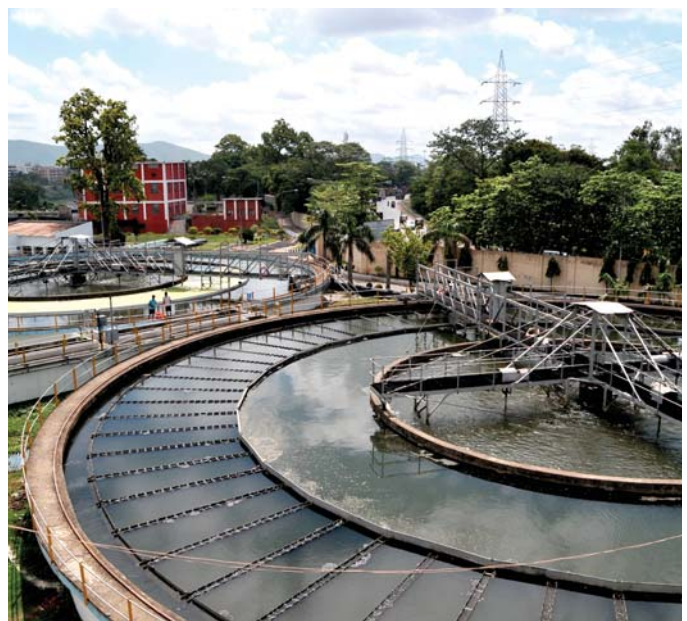
State of the art Waste Water Treatment plants at Jamshedpur
