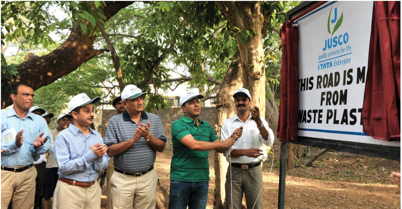
Waste plastic mixed with bitumen to build roads keep the city clean of plastics as well as strengthens its roads
