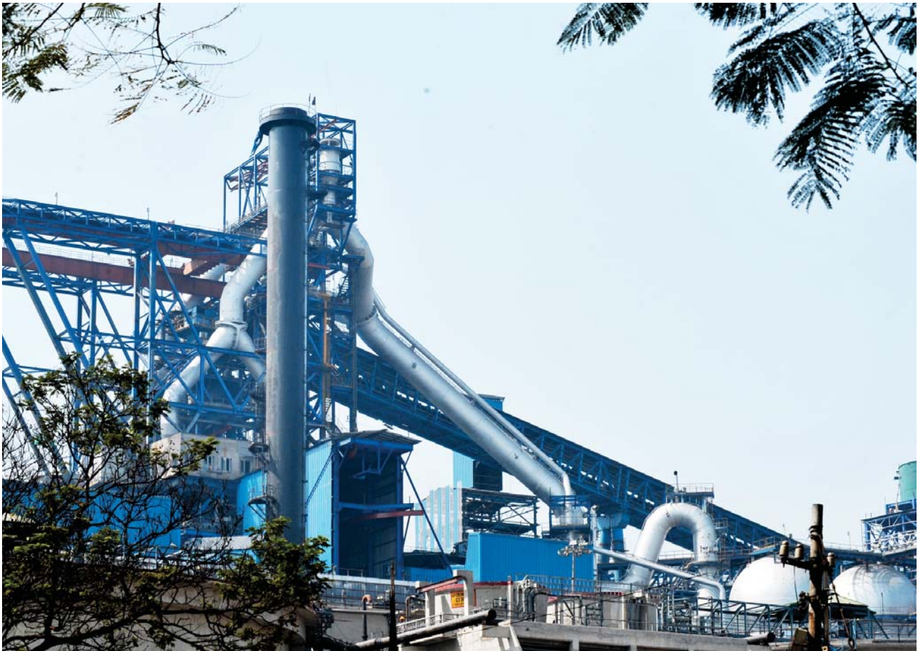
Dust suppression equipment at the Steel Works has improved overall air quality
