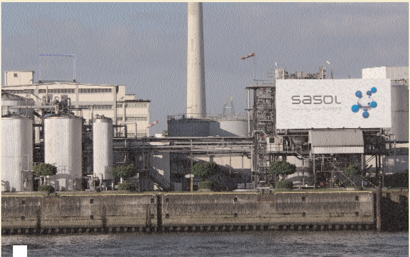
The Sasol Wax plant alongside the River Elbe at Hamburg, northern Germany. This business improved the performance of its steam-generation units and reduced carbon-dioxide emissions by 20%.
