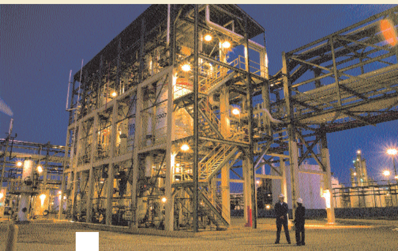
One of the manufacturing facilities at Sasol North America's Lake Charles chemical complex.
