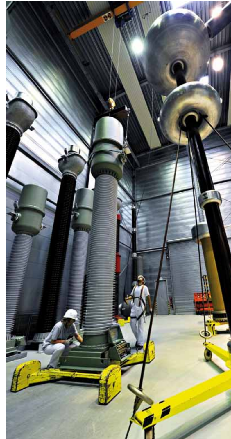
An instrument transformer at the Alstom site in Ludwigslust, Germany.
