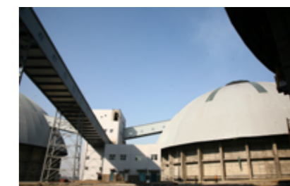
Closed raw material silo of Bayi Iron & Steel
