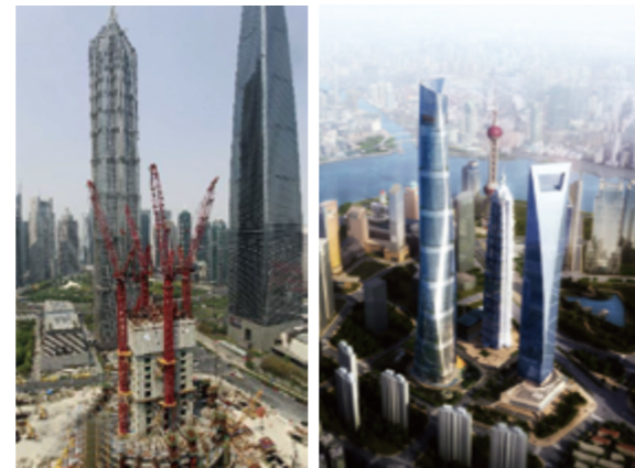
The construction site The presentation drawing
