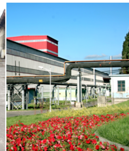
Landscaped plant area of Bayi Iron & Steel
