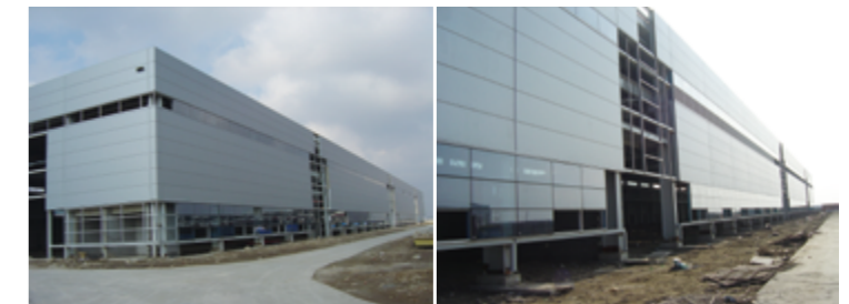
Production tooling plant Digital control plant
