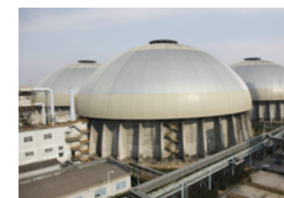
Closed raw material silo of Ningbo Steel
