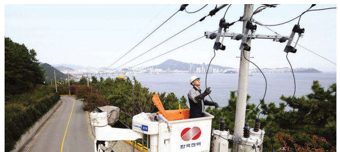
▶ electricity quality inspection
