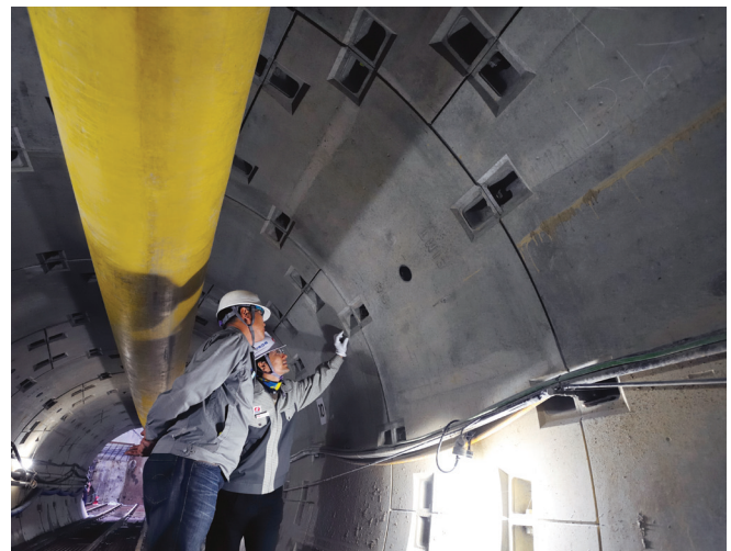
On-site safety inspection
