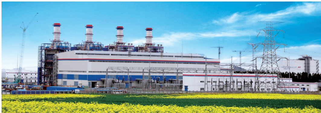
Putian Gas-fired Power Plant, the largest clean energy power plant in China
