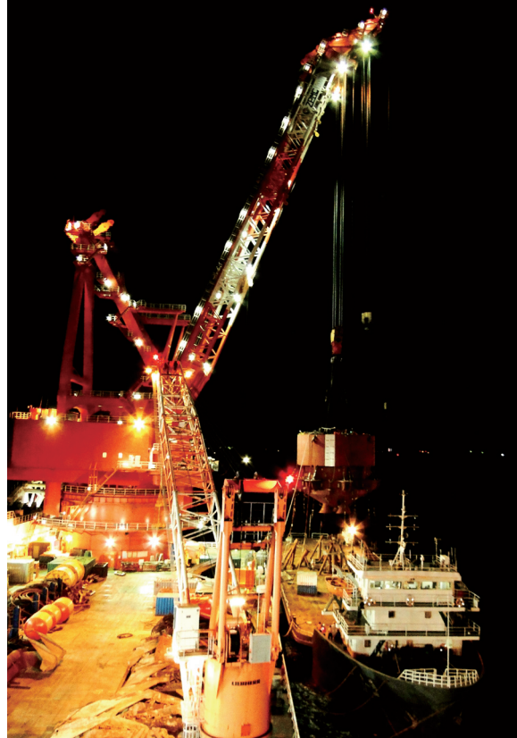
Offshore oil engineering service: Hoisting Operations
