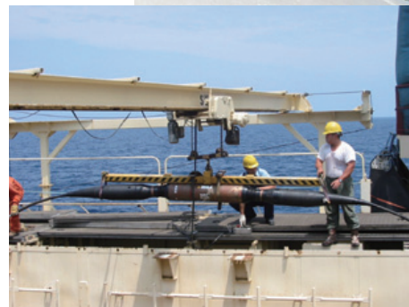
Installation of submarine cable
