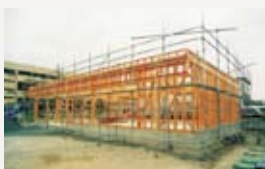
Store under construction
