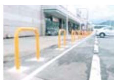
Parking Lot Guardrails
