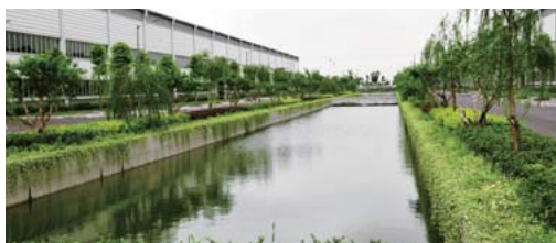
Pond where recycled water is stored after treatment
