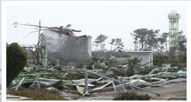
The tsunami wrecked pipes, wastewater intake equipment, pumping towers, machinery, and electrical equipment. Much equipment was destroyed.
