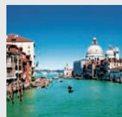
ArcelorMittal's steel sheet pile technology was chosen as the most efficient solution for the lock structures and for the foundations of the steel barriers to help preserve Venice from future floods.
