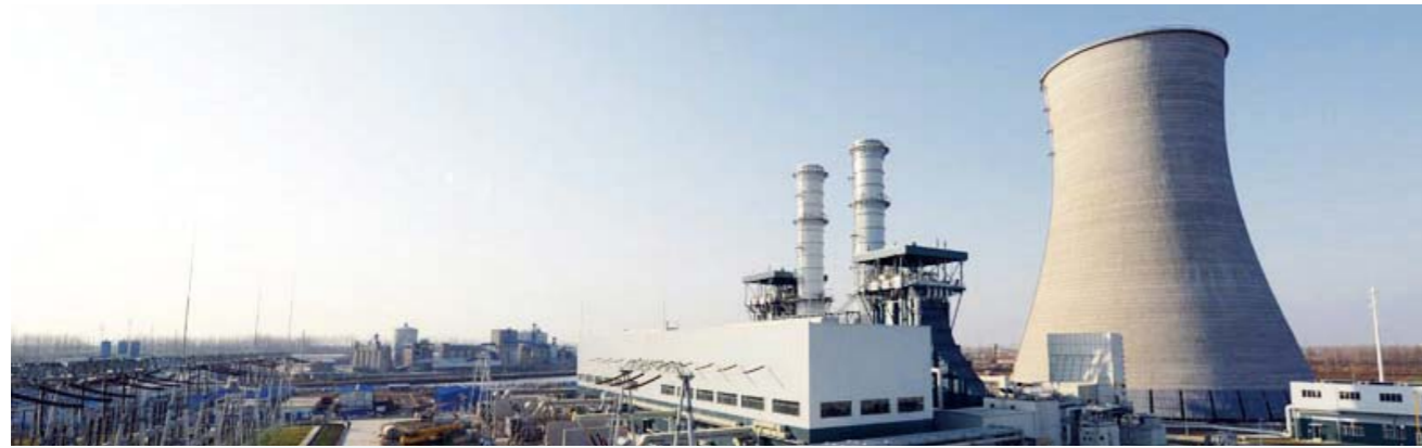
燃气电厂 Natural gas power plant
