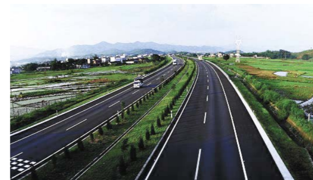
京珠高速公路 Section of the Beijing-Zhuhai Expressway
