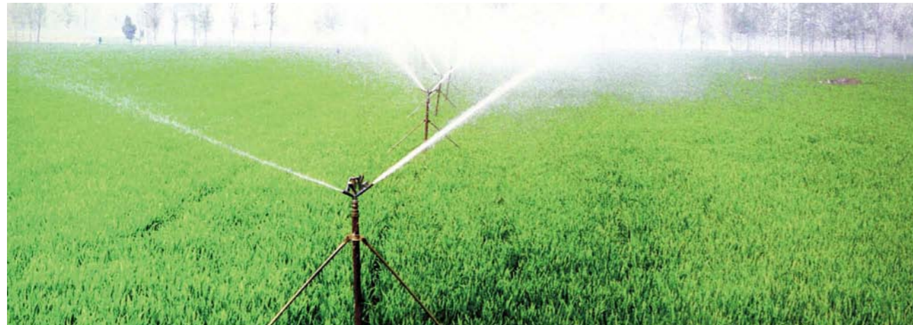
周口市农田节水喷灌系统 Water-efficient irrigation facilities in Zhoukou City
