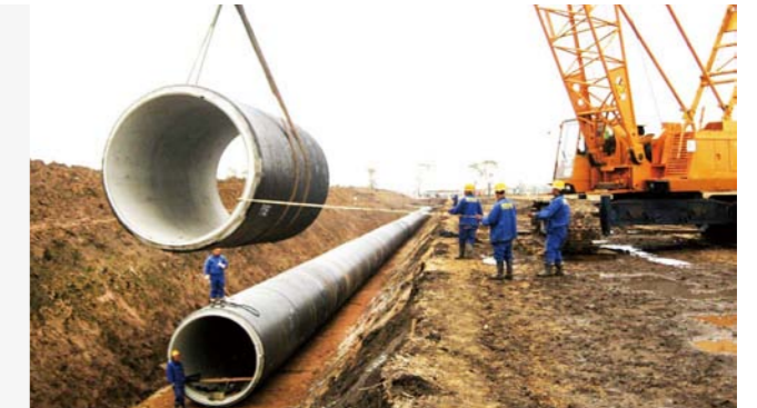
输水管道安装 Installation of water pipeline
