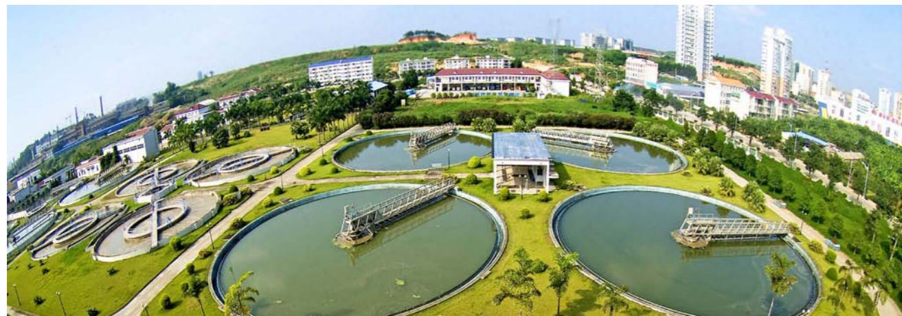
琅东污水处理厂 Langdong Sewage Disposal Plant
