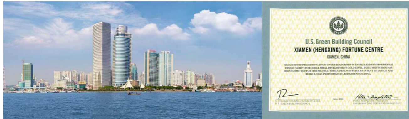
厦门分行办公楼远景图 A panoramic view of the office building of CDB Xiamen Branch
