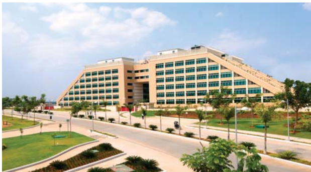
Energy-efficient building at the Pocharam campus, Hyderabad
