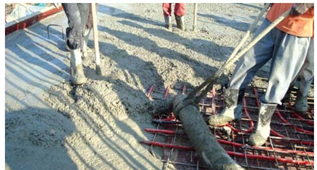
Slab casting with radiant cooling pipes
