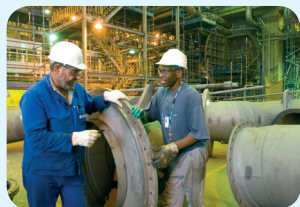
Restoration work at Komati power station
