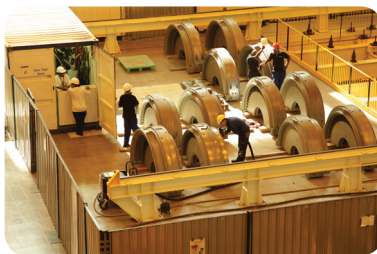
Maintenance work at the Koeberg nuclear power station
