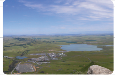
The Braamhoek dam is complete at the new Ingula pumped storage scheme
