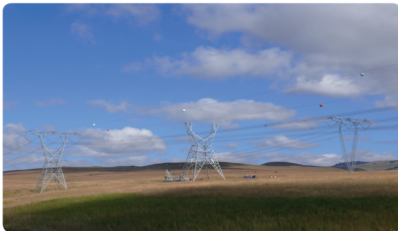
New high-voltage lines are erected from the Ingula pumped storage scheme near Ladysmith
