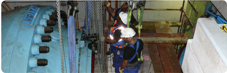
Maintenance at the Palmiet pumped storage scheme near Grabouw
