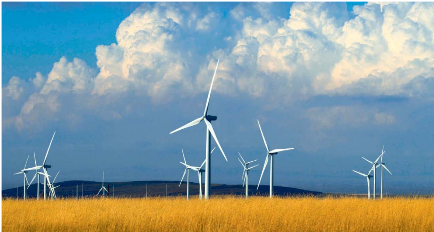
Goshen wind farm, Idaho, US
