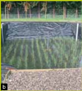
b A reed bed breaks down sludge from our Blair Athol malt whisky distillery in Scotland, reducing its environmental impact.
