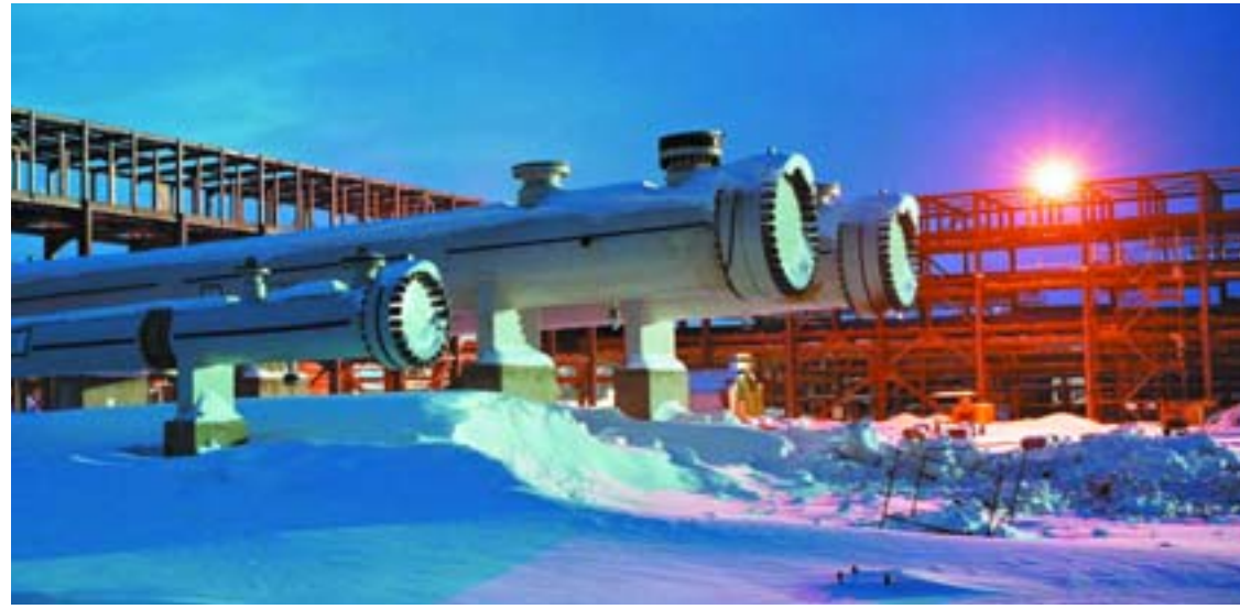
> HEAT EXCHANGERS AT THE ONSHORE PROCESSING FACILITY CONSTRUCTION SITE
