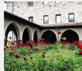
The cloister of the Eremo dei Ss. Pietro e Paolo a Bienno, restructured thanks to a donation from the Banca di Valle Camonica
