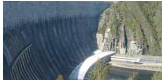
DAM OF SAYANO-SHUSHENSKAYA HPP
