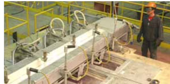
NEW CASTING LINE AT KRASNOYARSK ALUMINIUM SMELTER
