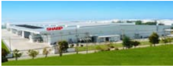
SATL's new Cool e 3 plant
