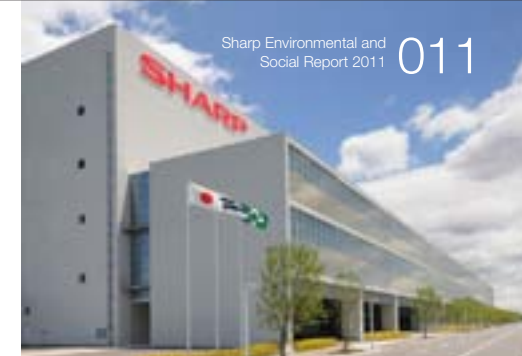
Solar cell plant at GREEN FRONT SAKAI
