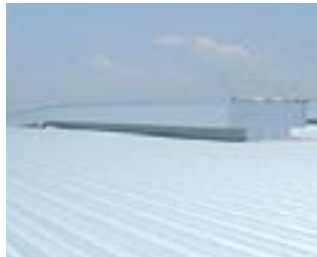
Air is sent out through a monitor roof
