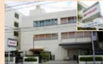
The current office building
