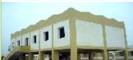
Community cum Flood Relief Centre
