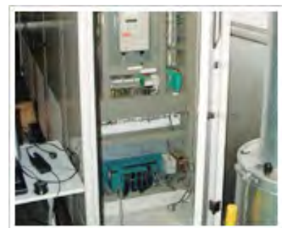
STARDOM controller installed in the site cabinet
