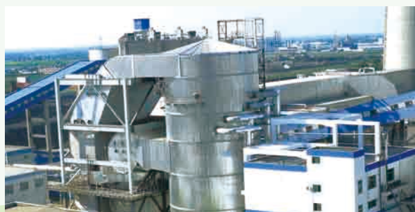
◆ Desulfurization system of Huaneng Dezhou power plant Phase 3 Project put into operation
