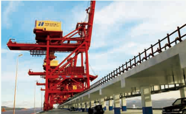
◆ Coal transportation dock of Huaneng Yuhuan Power Plant
