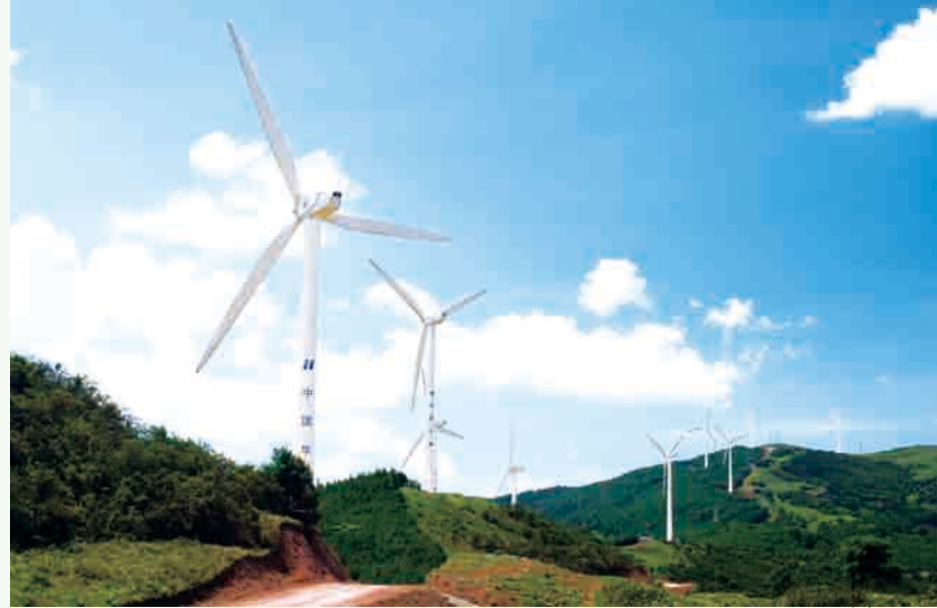
◆ Wind farm with the highest elevation in China- Huaneng & HK Electric Dali Dafengba Wind Farm.
