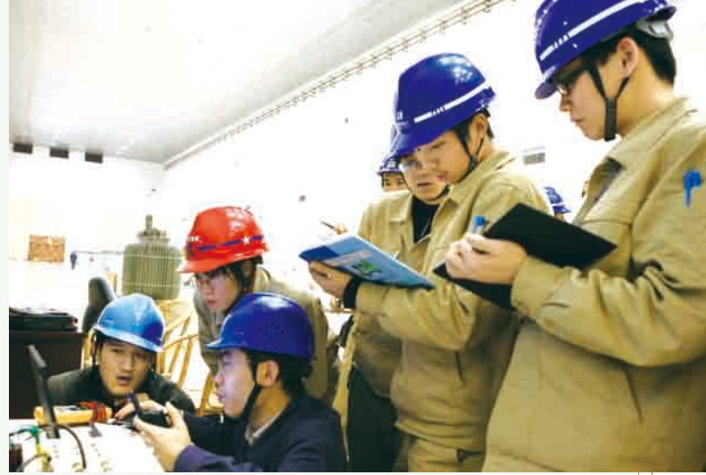
◆ Skill training on-site
