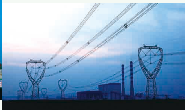
◆ Transmission network of Huaneng Shangdu Power Plant
