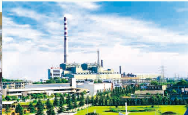
◆ Huaneng Yueyang Power Plant
