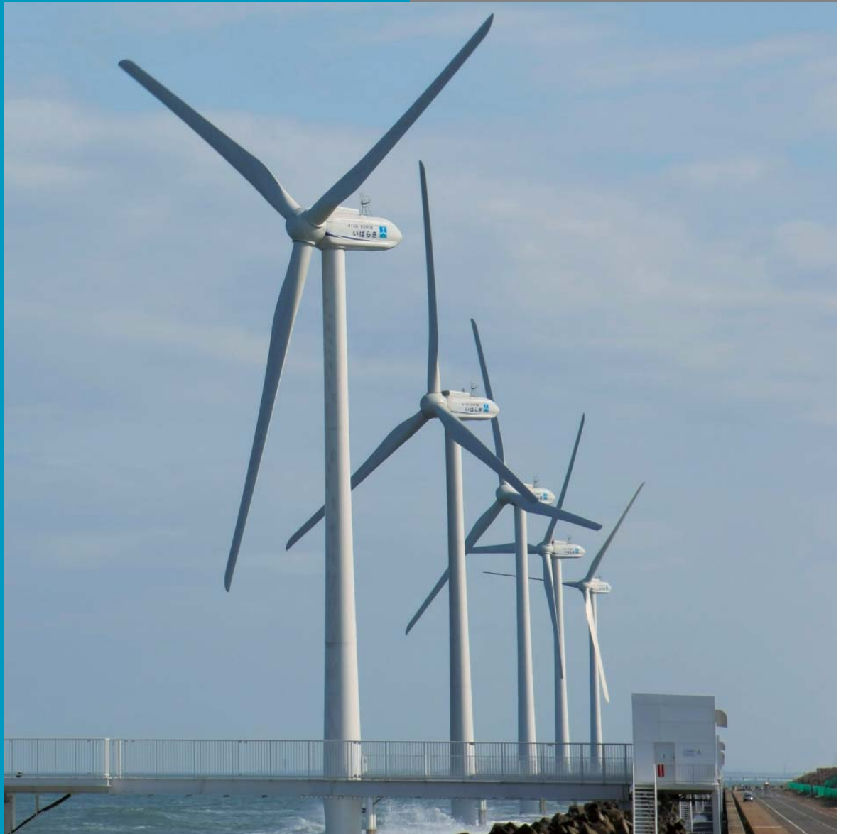
Wind Power Ibaraki Co., Ltd's Wind Power Kamisu (seven 2,000-kW wind power turbines)
