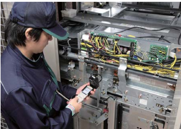
Maintaining an elevator control board
