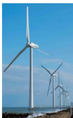
Wind Power Ibaraki Co., Ltd's Wind Power Kamisu
