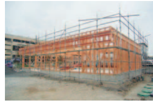
Store under construction
