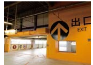
Large direction signs in multi-story car parks
