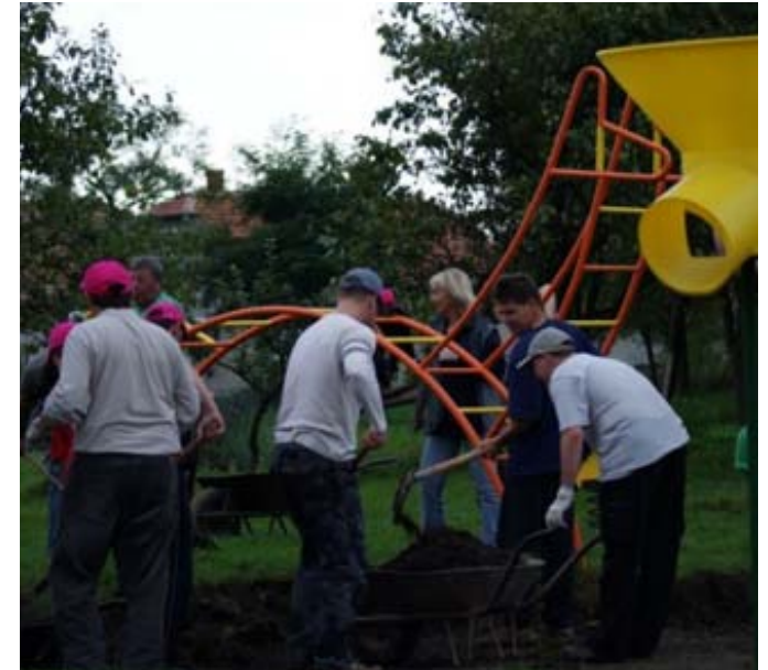
Kindergarten renovation in Gelej – Telekom voluntary team building
