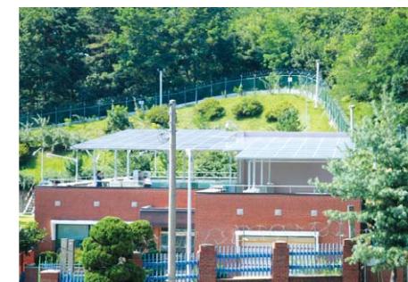
- Photovoltaic power generation facility
