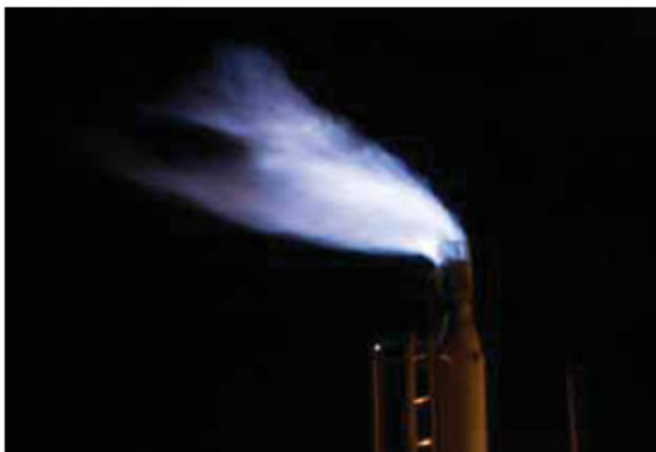
The underground coal-gasification flarestack with Majuba power station in the background (blue flame typical for UCG gas).
