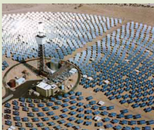
Concentrating solar plant to be built near Upington in the Northern Cape.
