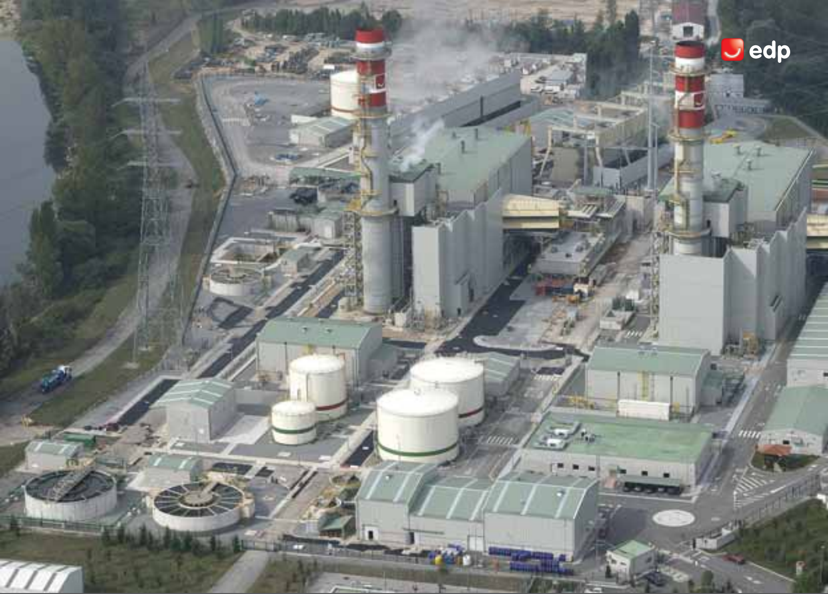
Soto Ribera – Soto 5 combined cycle gas turbine
