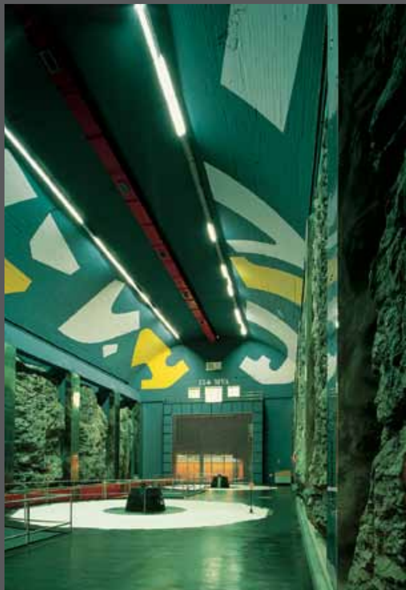
Tanes Hydroelectric Power Plant
