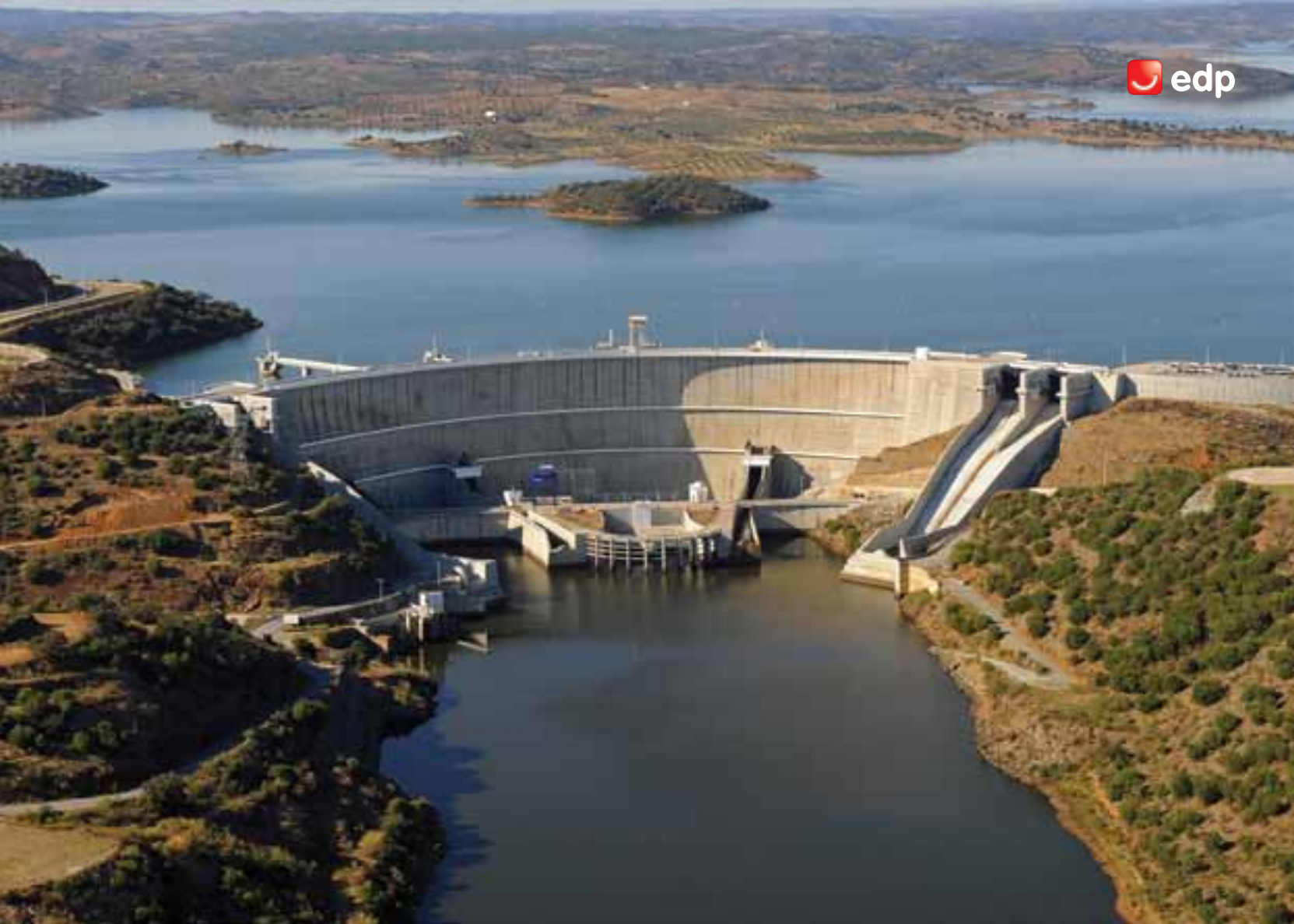
Alqueva Hydroelectric Power Plant
