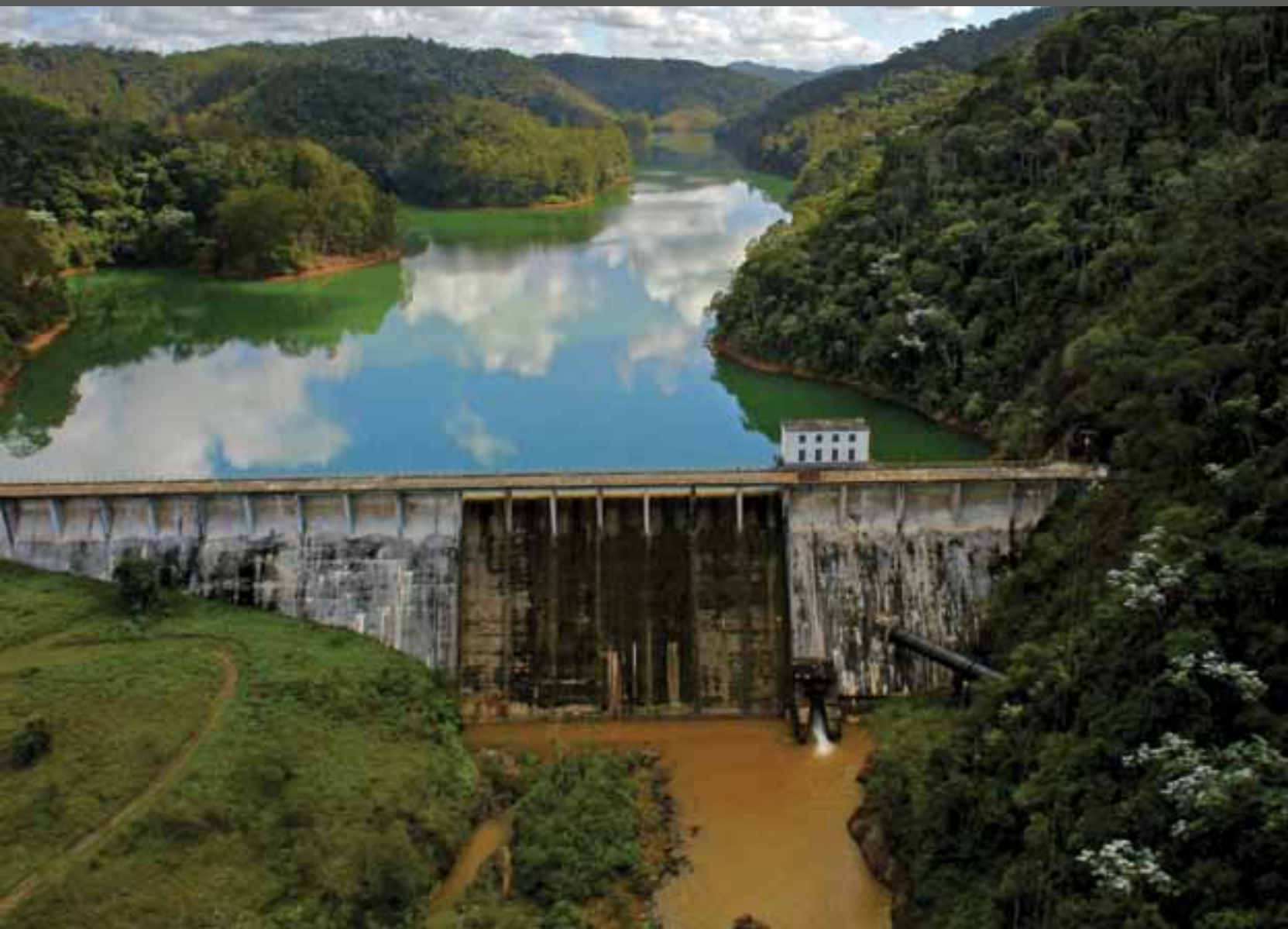
Rio Bonito Mini Hydroelectric Power Plant
