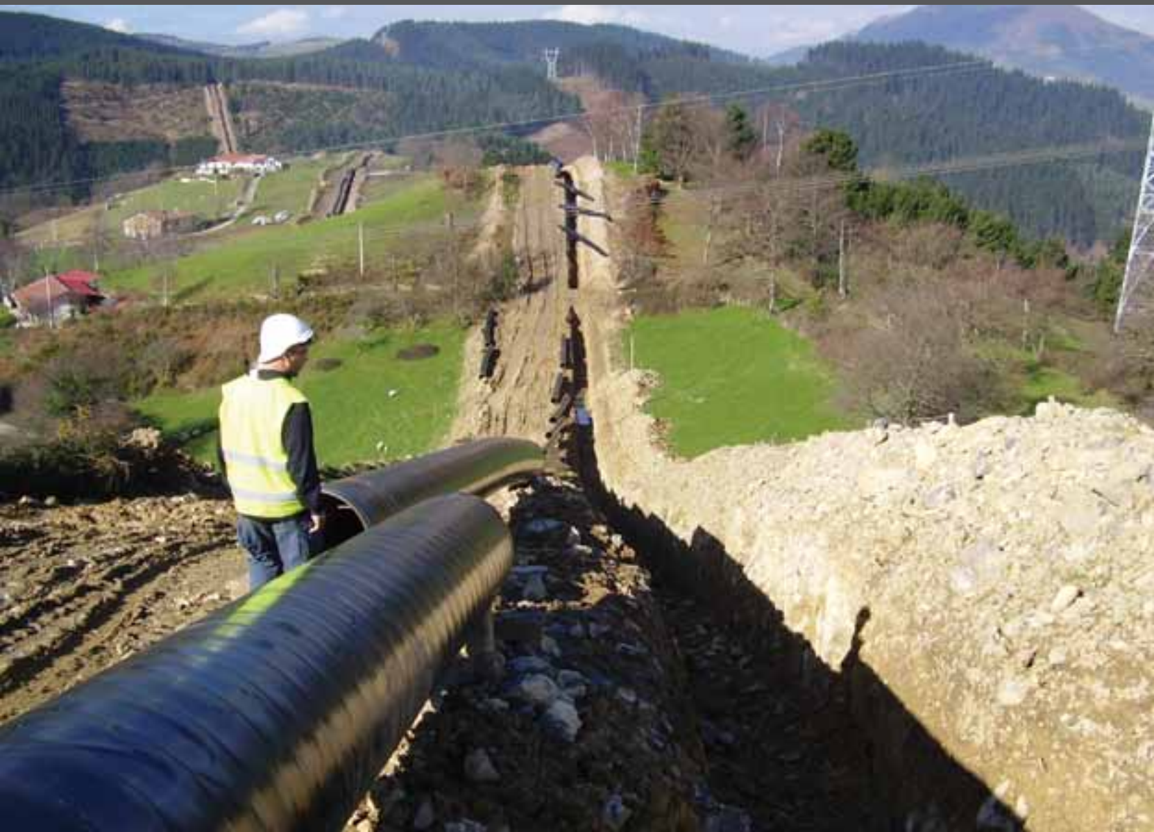
Bergara-Irún Gas Pipeline
