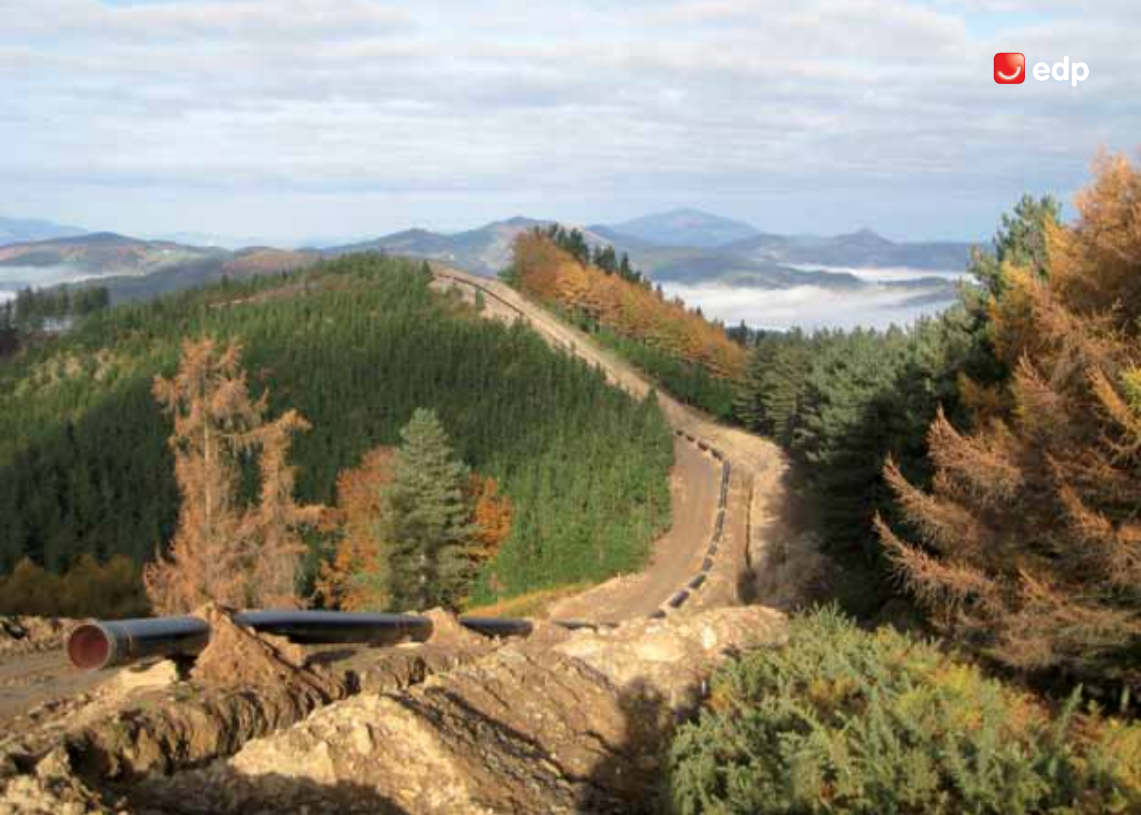
Bergara-Irún Gas Pipeline
