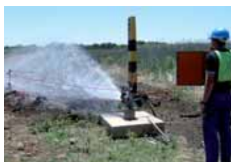
Pump testing a new borehole in the Vaal River area to determine the volume of water that can be pumped on a daily basis
